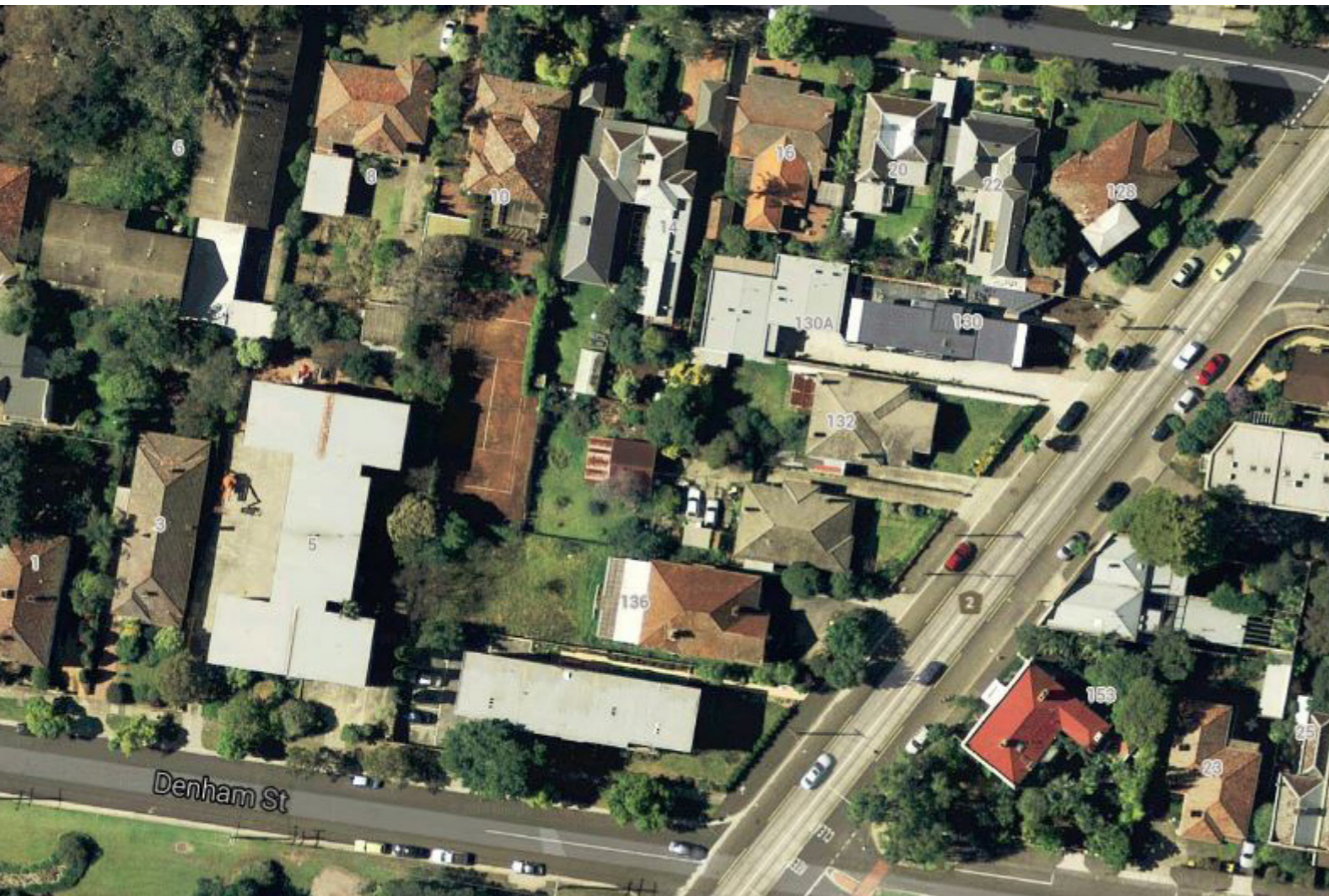
Figure 4: Aerial photo, predating the redevelopment of no. 136 Church Street, showing the primary and secondary area considered relevant.
