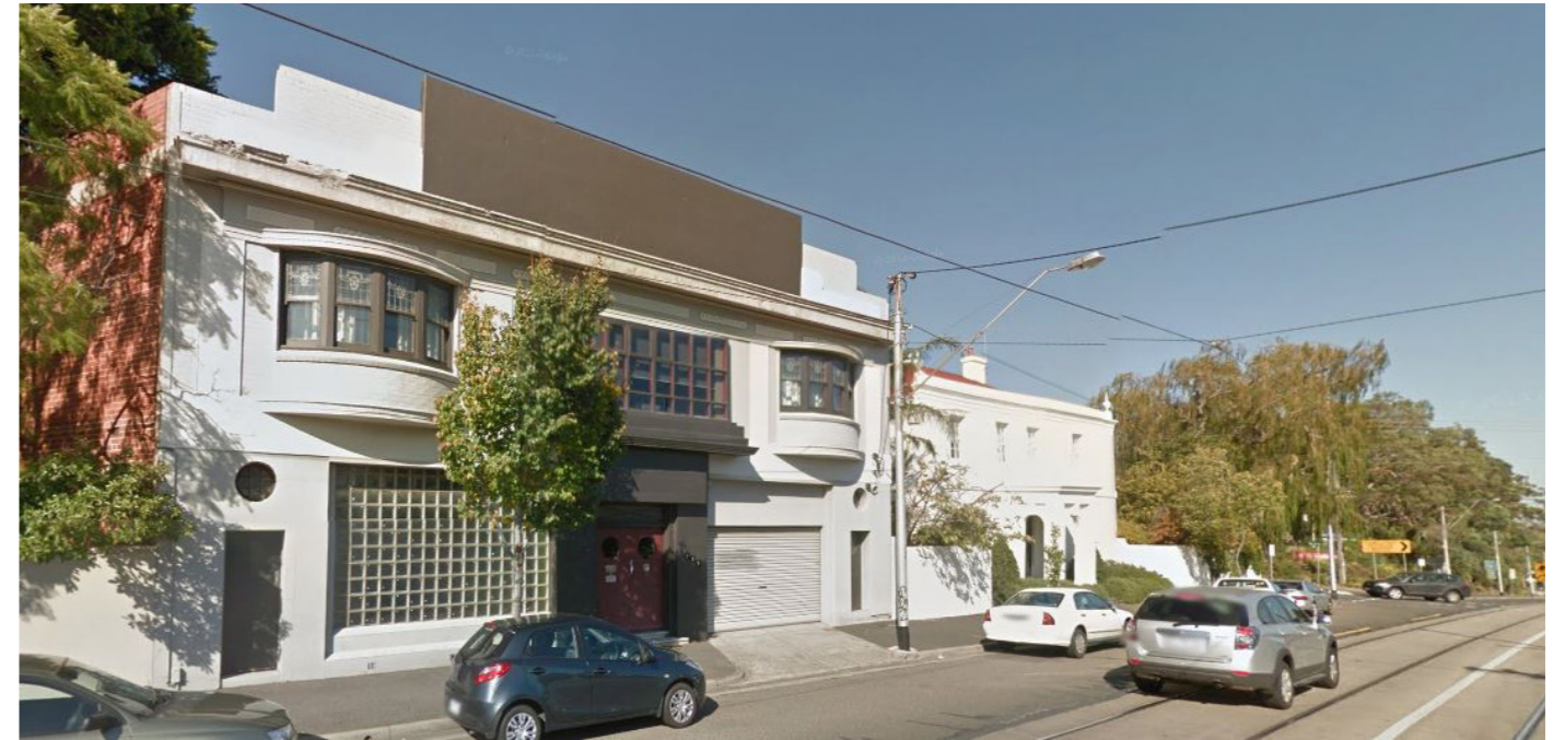
Figure 3: View from the street of no.s 153 and 155 Church Street
